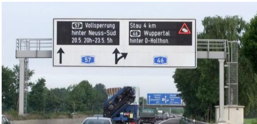
**Figure 1 – dWiSta: dynamic sign post with integrated traffic information [THOMAS Verkehrstechnik]**
